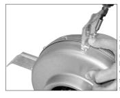
3. Fasten the mounting brackets with the self-drilling screws.
