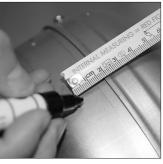
2. Mark the measure of C. Start from the joint of the fan.
